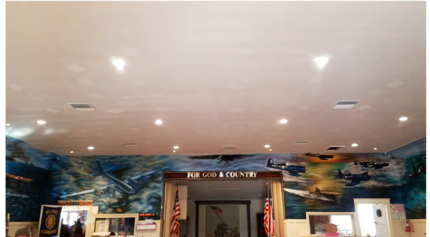
Above: The finished ceiling: with new LED lighting, drywall, and paint.
